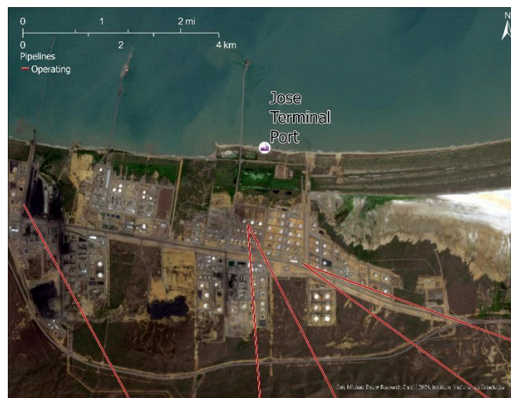
Figure 2. High-resolution PlanetScope imagery of the José Industrial Complex showing pipeline connections, crude oil storage tanks, loading berths, and export infrastructure. Source: Planet Labs PBC, PlanetScope imagery, March 1, 2026.
